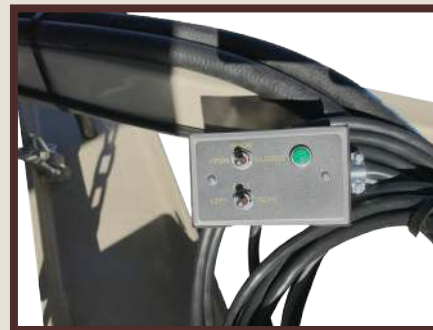
Momentary switch for hydraulic trap door and conveyor belt
